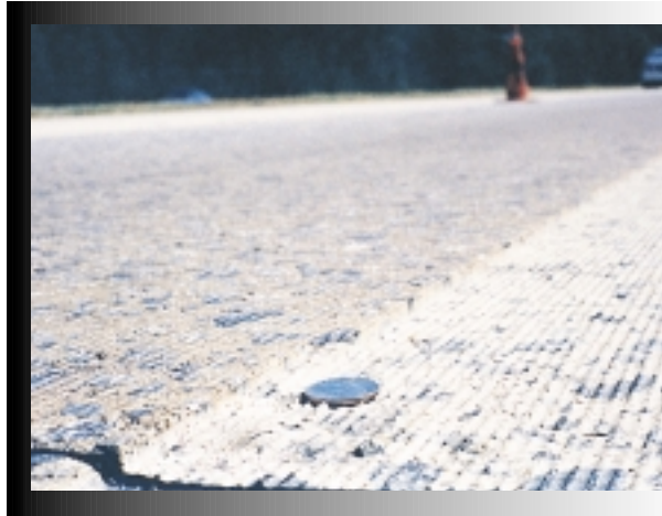
A close-up of diamond-ground concrete pavement shows the surface texture. (69075)
